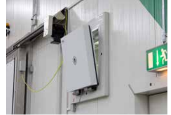
Pressure equalisation hatch for stabilising flexible doors panels.
