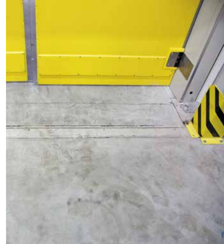
Heated floor area and adjacent mating door seal
