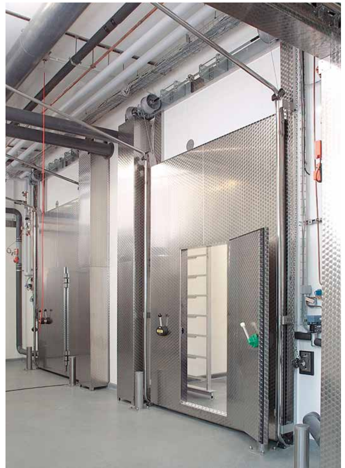
Precise planning and installation of V2A lift gates.
