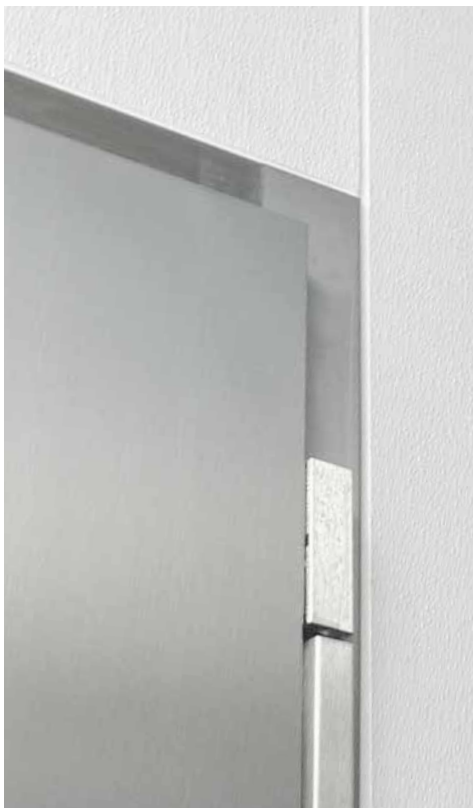
Flush door frame installation
