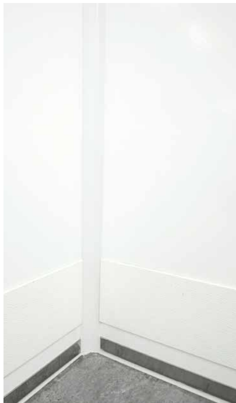
GRP elements with rounded inner corner and GRP impact protection
